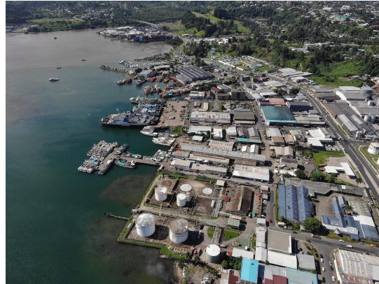
Muaiwalu I & II Local Wharves Rehabilitation (Construction)
