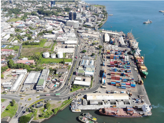
Port of Suva Capacity Enhancement (Phase 1 & 2)
